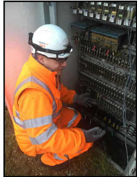
Image courtesy of Network Rail https://www.networkrailmediacentre.co.uk
