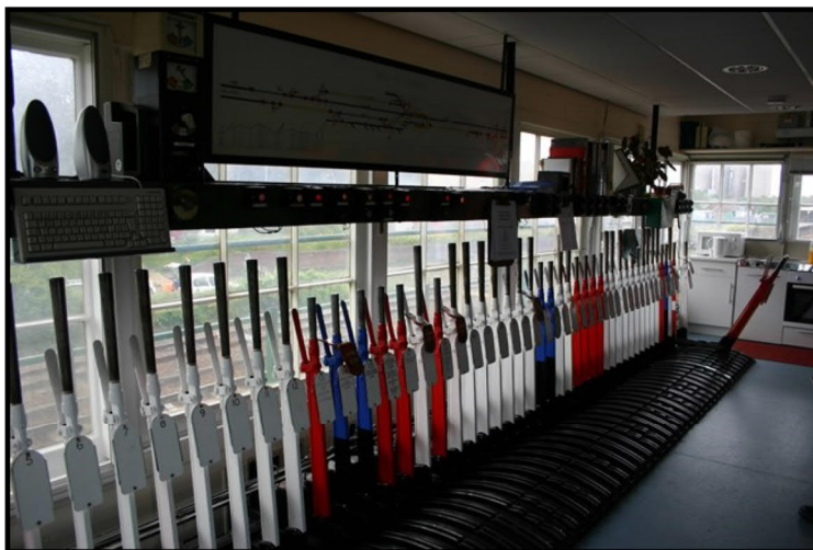
Image courtesy of Network Rail https://www.networkrailmediacentre.co.uk
