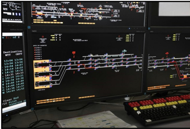
Image courtesy of Network Rail https://www.networkrailmediacentre.co.uk
