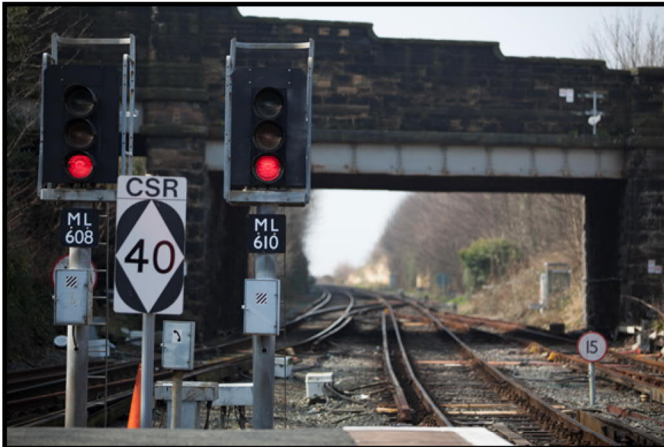
Image courtesy of Network Rail https://www.networkrailmediacentre.co.uk
