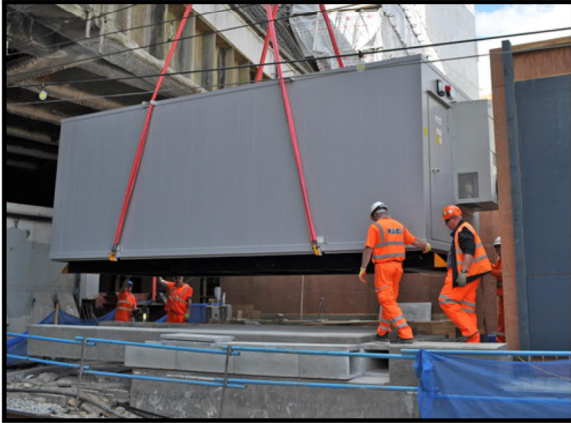
Image courtesy of Network Rail https://www.networkrailmediacentre.co.uk
